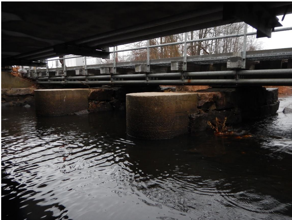
Looking downstream. Note redone pier sections (GSE; 12/17/2015)
