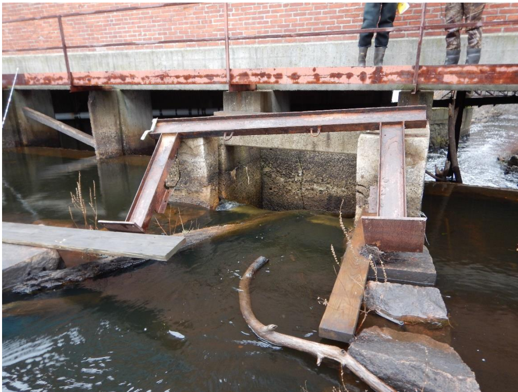
Looking downstream at the low-level outlet (GSE, 12/18/2015)
