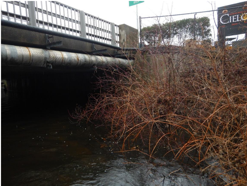
Looking downstream toward the right bank (GSE, 12/17/2015)
