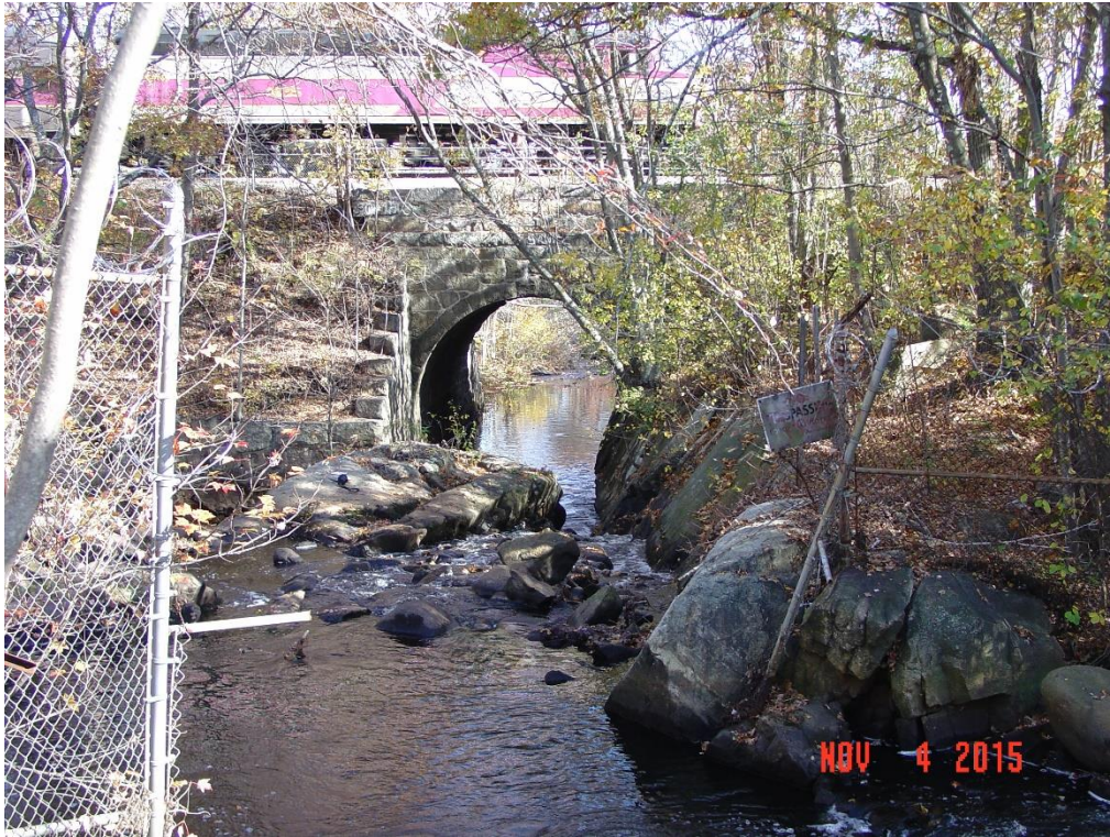
Photo 1: Downstream MBTA Railroad Bridge
