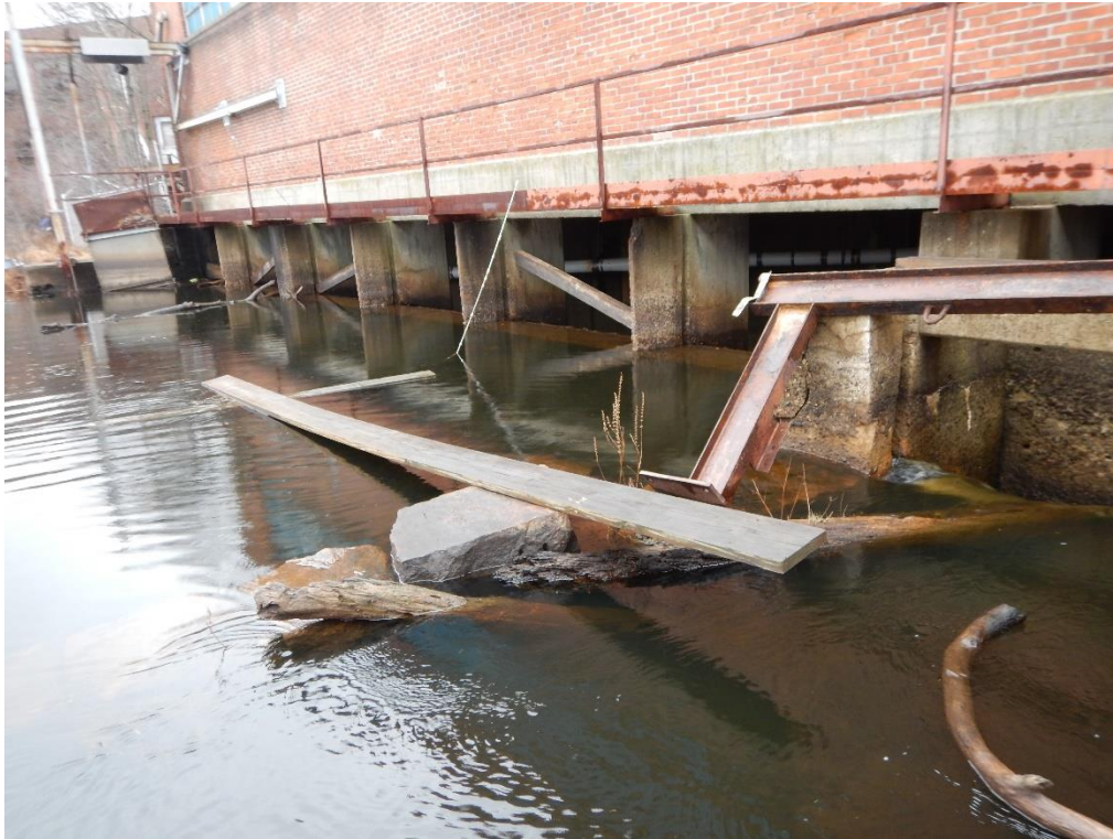
Looking downstream at Armstrong Dam gates and catwalk (GSE, 12/18/2015)
