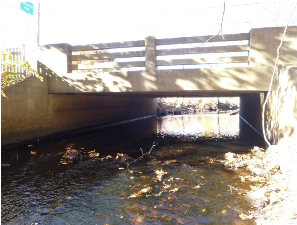
Facing upstream at the Jefferson Street Bridge (GSE, 11/03/2015)
