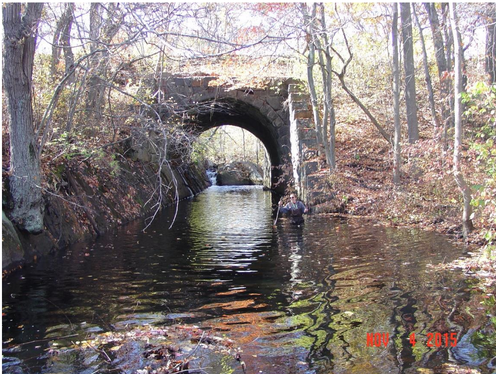
Photo 2: Downstream MBTA Railroad Bridge
