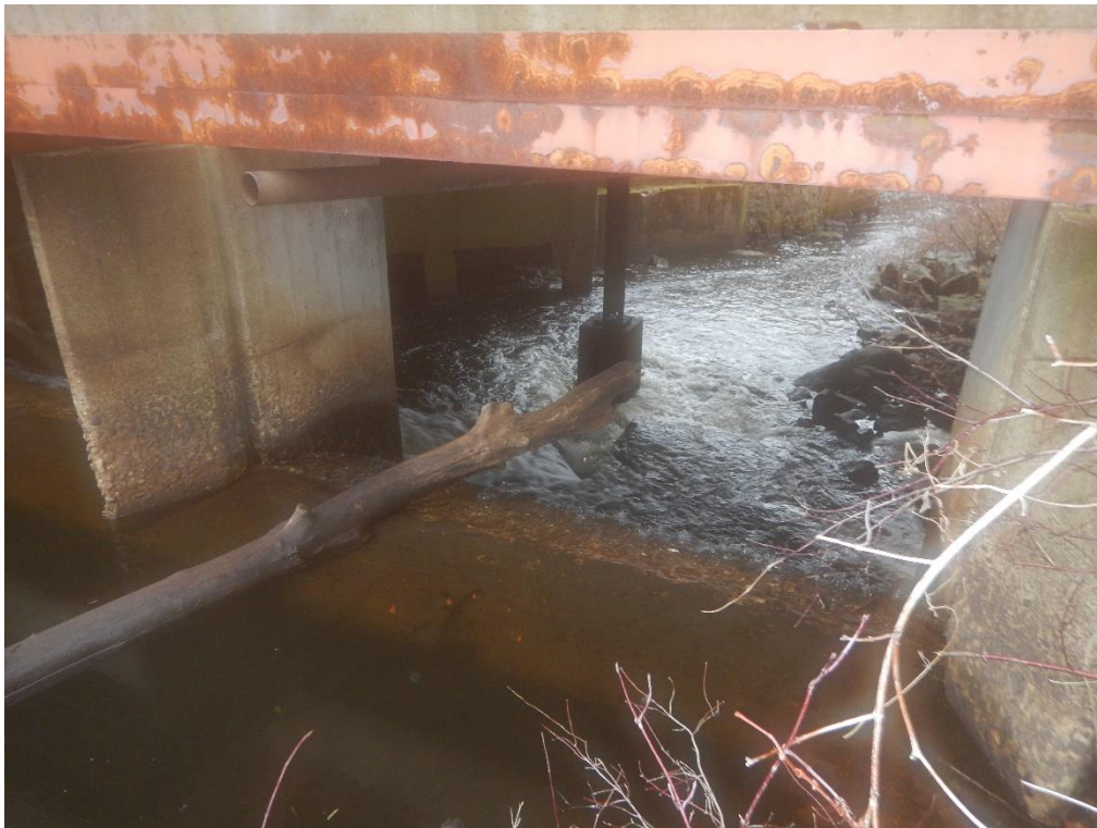
Looking downstream from the front of Armstrong Dam (GSE, 12/18/2015)
