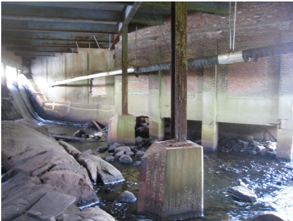
Looking at structural supports from river right (GSE, 07/09/2008)
