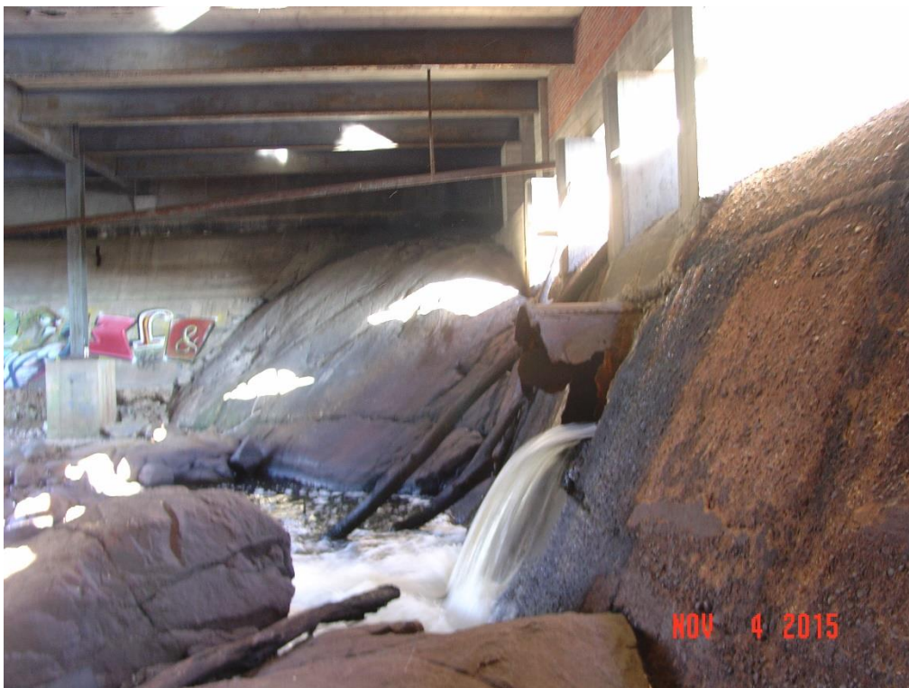
Looking toward river right bank/abutment (GSE, 11/04/2015)
