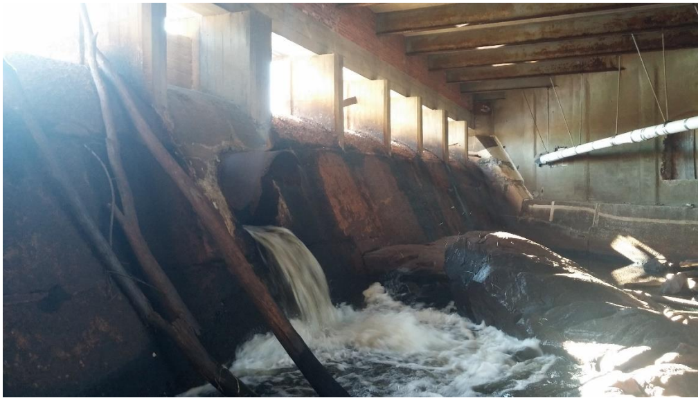
Looking toward river left bank/abutment (GSE, 11/04/2015)
