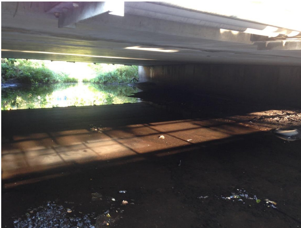
Facing upstream from right bank (GSE; 09/08/2015)
