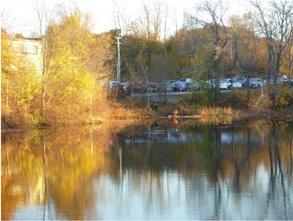
Looking upstream from the catwalk above the Armstrong Dam (GSE, 11/04/2015)
