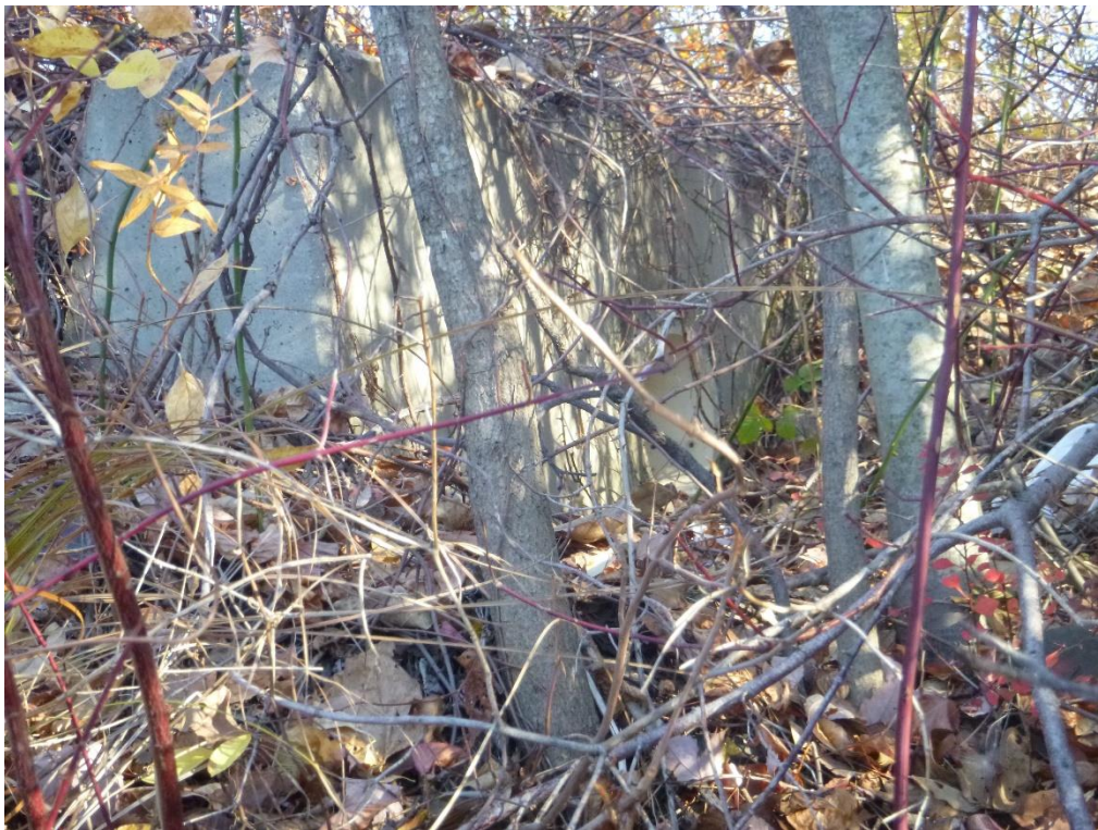
Looking downstream toward the left bank (GSE, 11/03/2015)
