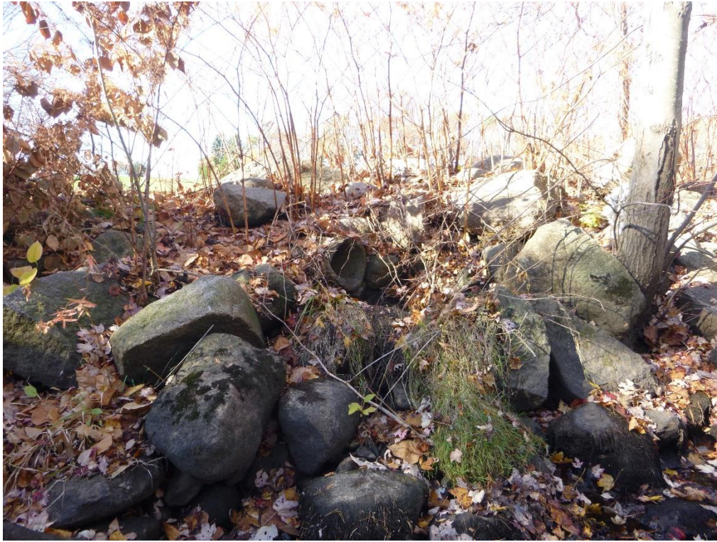
Looking downstream toward the right bank (GSE, 11/04/2015)
