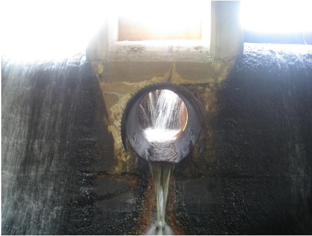
Looking upstream at the low-level out discharge culvert (GSE, 07/09/2008)
