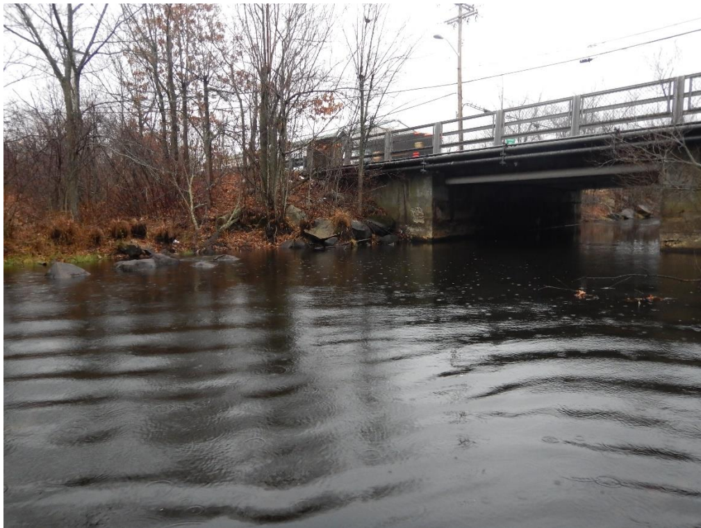
Looking upstream toward right bank (GSE, 12/17/2015)
