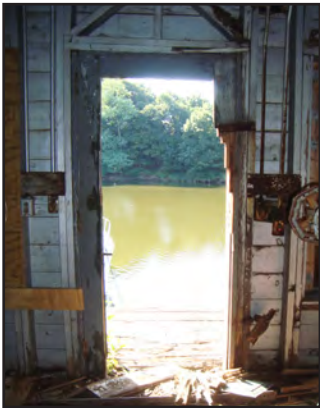
Above: The Screen House, located on the southwest portion of the site, has a cantilevered concrete walkway that extends out over the Monatiquot River.
