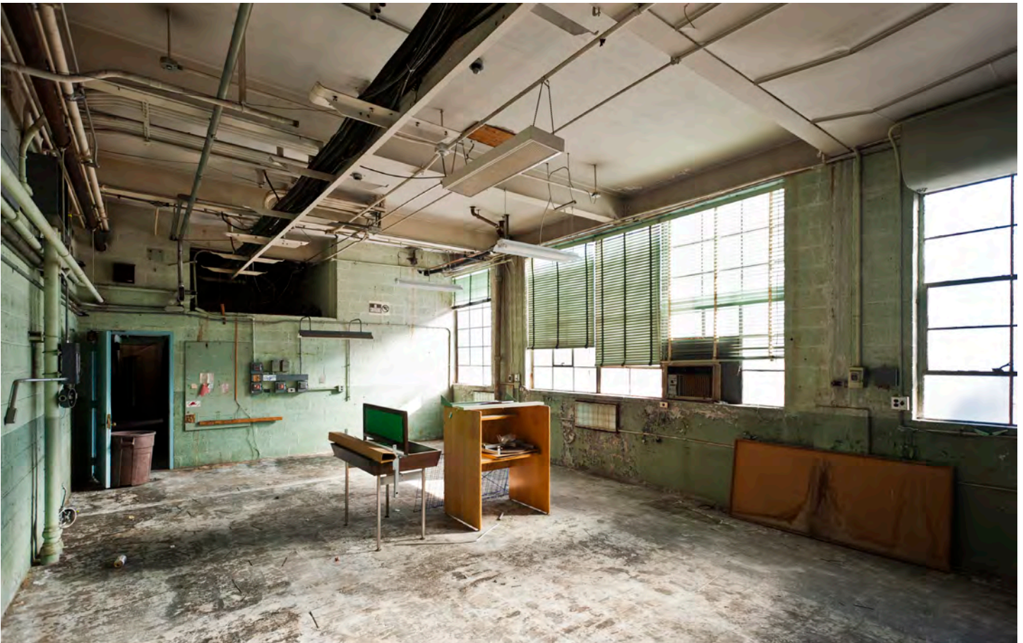
Top: Existing images of the Monaquot River and the Screen House (left), the former Administration Building (center), and the Switch House (right). Above: Lower level of the Switch House.
